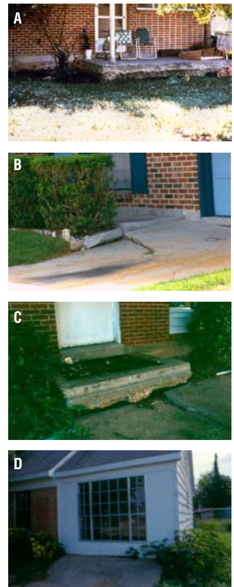
Figure 3. New Orleans area homes showing surficial subsidence effects ultimately resulting from the fact that the homes were built in an area of wetland soils. Alterations of the ground and its surface drainage have led to dewatering of clay and peat layers and oxidation of organic matter in the soil, the volume of which has shrunk dramatically over a period of just a few decades. The homes are on slabs atop pilings; the homes therefore do not sink as much as the surrounding ground. (Photo credits: A, J. O. Snowden, Southeast Missouri State University; B–D, Don Davis, Louisiana Oil Spill Coordinator’s Office.)
